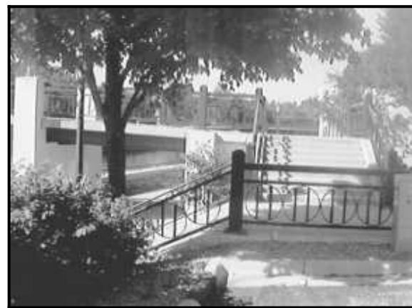
Figure 27 The Druid Bridge over the Cannon River in downtown Northfield with over 165 Druid Sigils on its railings, Summer 2004.
